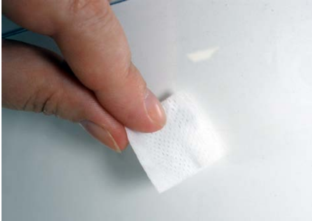
Figure 11. Adhesive Mount Antenna – Step 1. Pre-clean the surface
